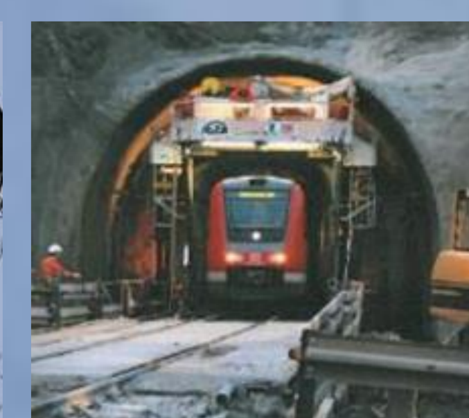
Figure 4: Tunnel bore widening
